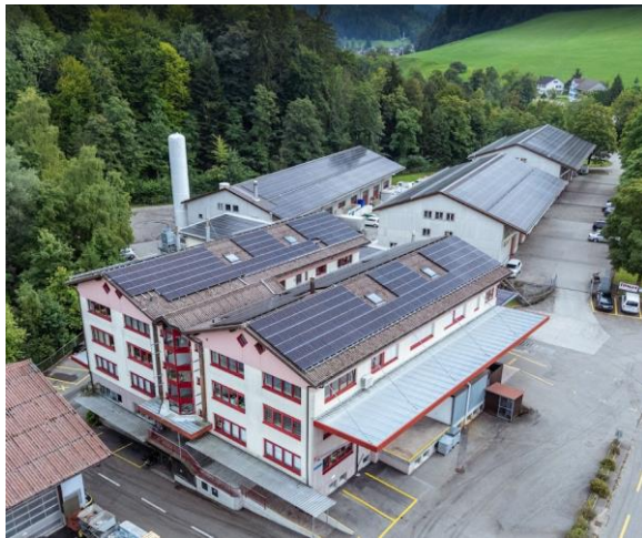
Figure 2: Aerial view of the Parmaco AG premises after installation of the photovoltaic system, showing fully integrated solar panels on the roof surfaces.
